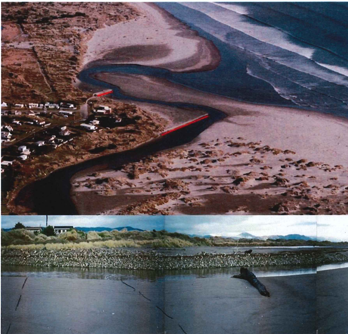
Figure 6: Upper photo (1996) shows the rock groynes (underlined red) that were constructed in 1991. Note the down-stream accretion behind each groyne. Lower photo shows the throat groyne in July 1994. Note the new dune development on accreting land on the far side of the groyne. (Source: kindly provided by Mr John Hewitson, Waikawa Beach).
