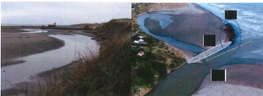
Figure 8: The most recent mouth cuts. Left photo taken on 10 July 2013 (source HRC), and right photo taken on 31 July 2018 (source HDC) shortly after the mouth cutting operation. Note in both cases the pre-diversion channel was against/close to the dune line at the back of the inlet. Note we were unable to source the original HDC photo so included the one above with various annotations unrelated to this study.
